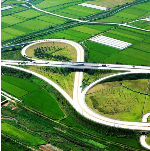
Asan Cheonan Expressway South Korea
